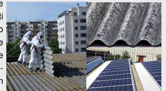
Coperture in amianto
